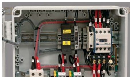
DIN rails for equipment or terminals with clip-on mounting
